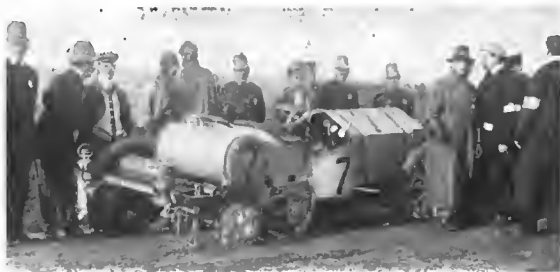
Acme After Its Drive Through the Fence.
